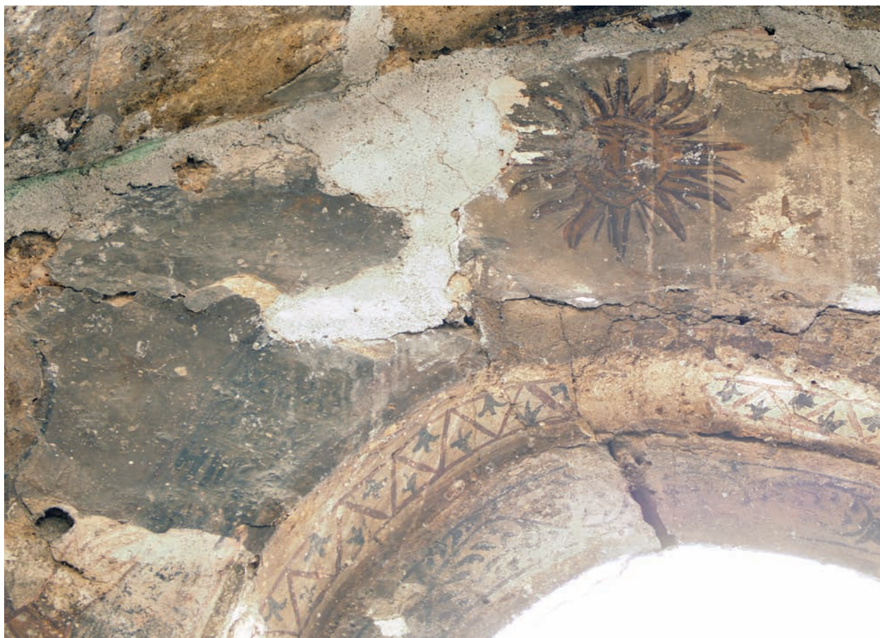
FIG. 42 Kazafani, Panagia tou Potamou, detail of the Last Judgment with detached plaster, damaged previous patching and algae growth. (Photo by T. Kaffenberger, 2016.)
