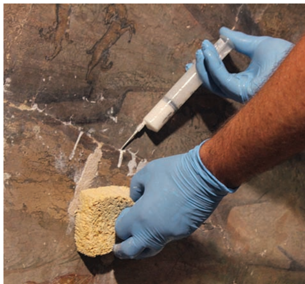
FIG. 43 Kazafani, Panagia tou Potamou, emergency stabilization: grout injection. (Photo by W. Schmid, 2017.)
